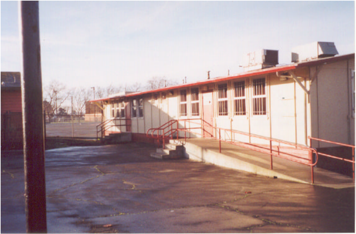
Figure 5: Rear of Main Building
