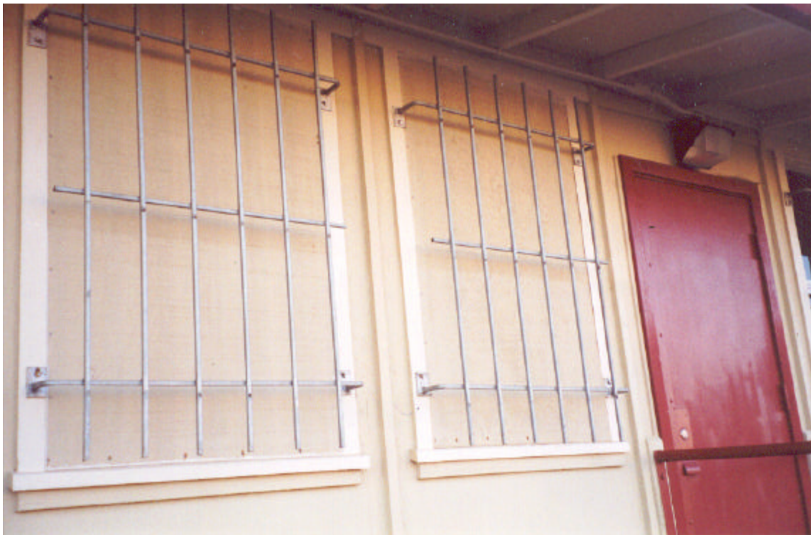
Figure 3: Plywood Window Infill at Front of Main Building
