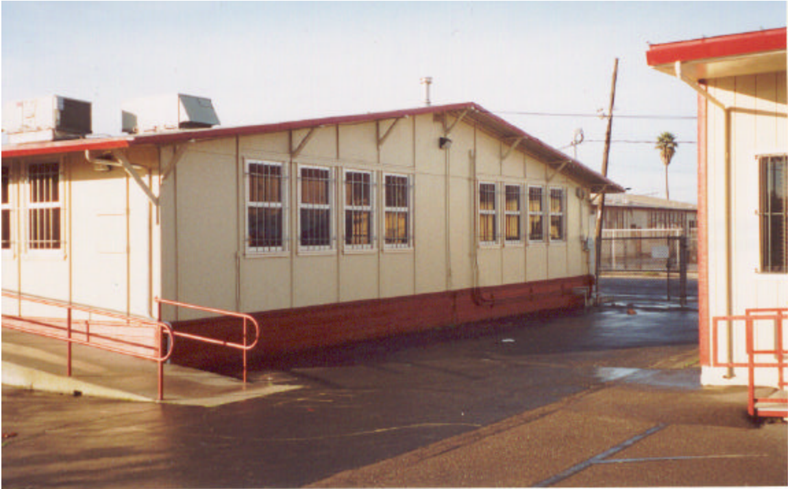
Figure 4: Side of Main Building
