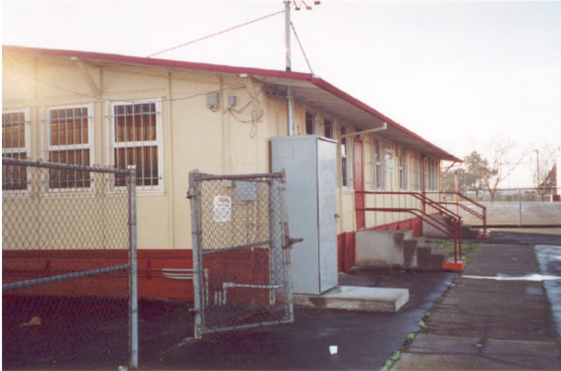
Figure 2: Front and Side of Main Building
