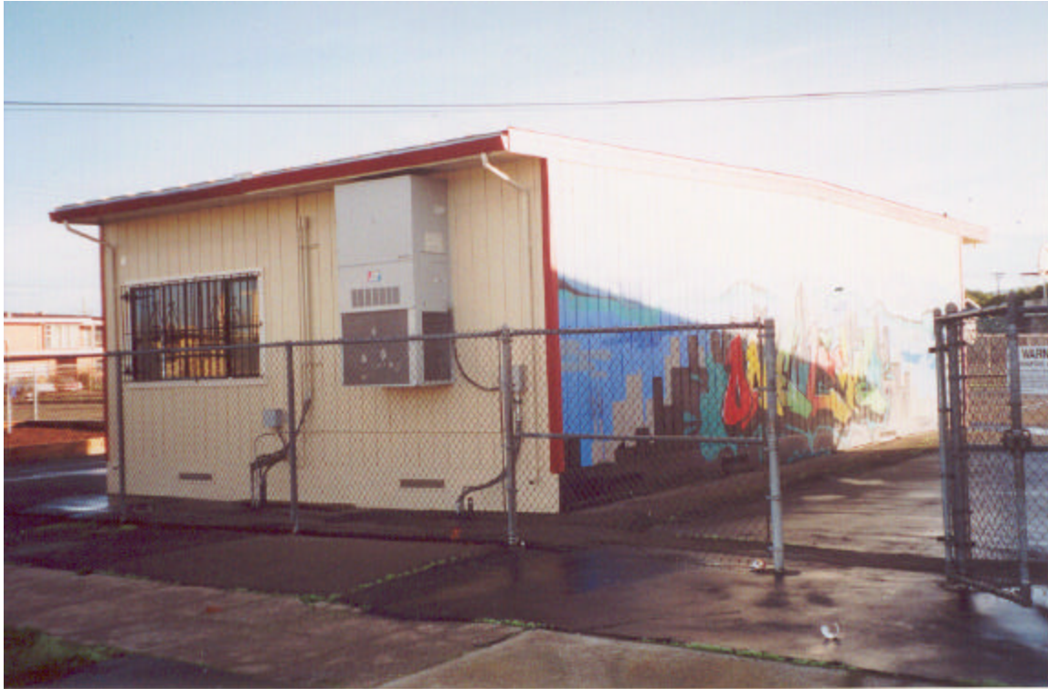
Figure 8: Side and Rear of Classroom Portable
